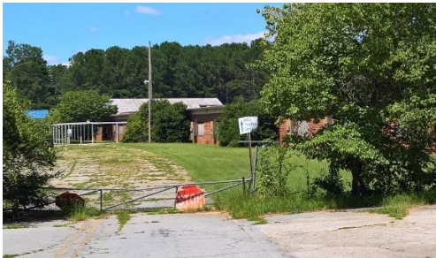
Old Henderson Mulberry Propriety when purchased in 2019 to Be Transformed into Community Workforce Development Center
